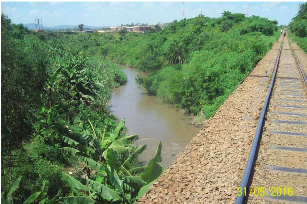
Plate 7: River bank encroachment along River Malaba in Malaba Town Council
