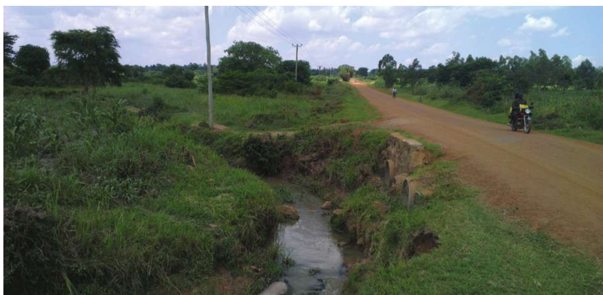
Plate 1: Soil erosion hot spot in P’Okongo bridge along Tororo-Nagongera-Busolwe road.
